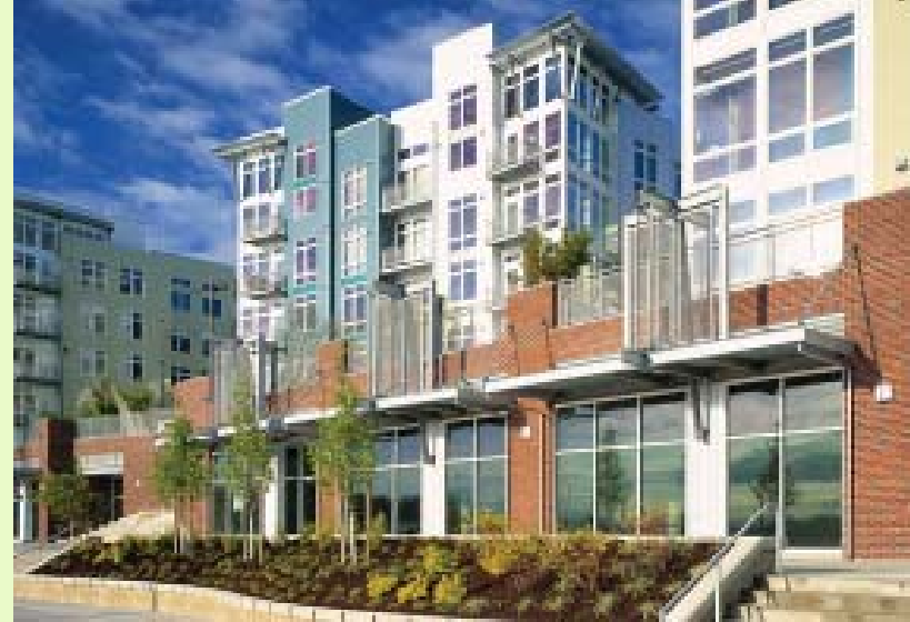
6 Story Buildings Set back from Parkway
